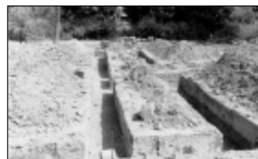
Not an archaeological dig, but the foundations of the future school and clinic.
